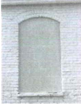
Removal of Boarded Windows
