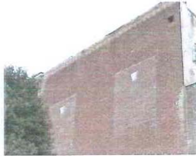
Removal of Bricked-up Windows
